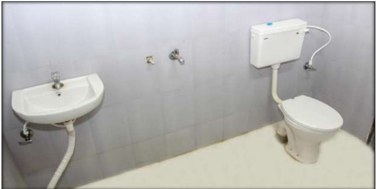
Restrooms for Divyangjan.
